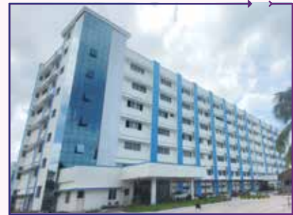
District Hospital, Mavelikkara Built-Up Area -2,16,670 sft (G + 4) Project Cost : ₹93.74 Cr
