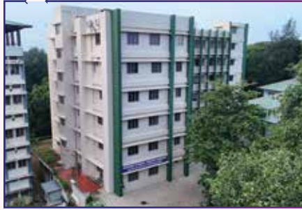
Government Medical College, Thiruvananthapuram, MLT Block Built-up Area – 46,242sft ( GF + 5 Floors) Project Cost : ₹18.90 Cr
