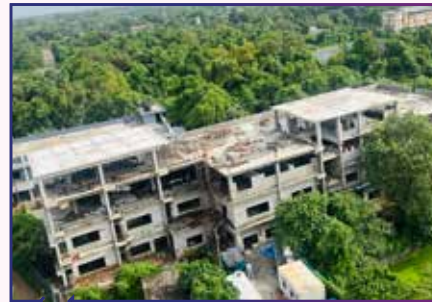
Critical Care Block at Government Medical College, Thirssur Built-Up Area - 42,740 sft Project Cost : ₹13.38 Cr
