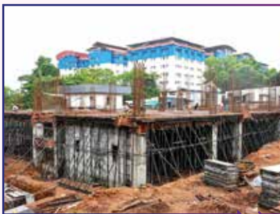
Critical Care Block at Government Medical College, Kannur Built-Up Area - 46,373 sft Project Cost : ₹16.38 Cr
