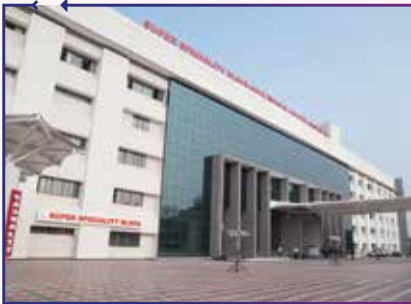
Government Medical College, Ernakulam Super Speciality Block Built-up Area – 8,27,000sft (LG - 3 Floors + GF + 4 Floors) Project Cost : ₹262 Cr
