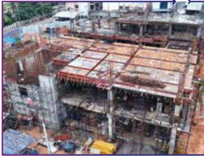
Government Medical College , Thiruvananthapuram - OT Block Built-Up Area - 1,47,375 sft (LG + G + 5) Project Cost : ₹81.56 Cr
