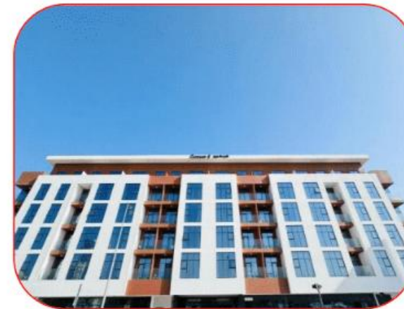
Sunday Sheikh Zayed Road Concord Tower, Dubai – 185 Keys
